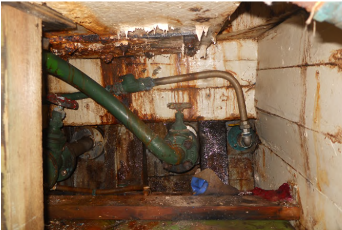
Engine Room 2.JPG
