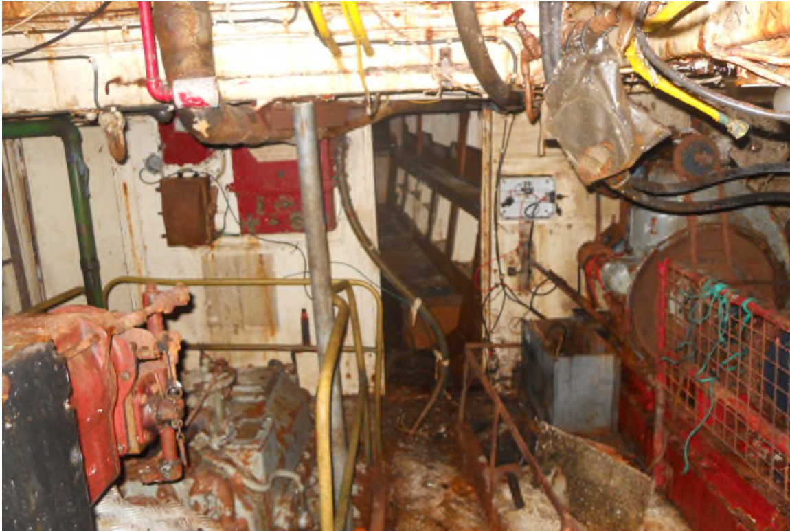
Engine Room 5.JPG
