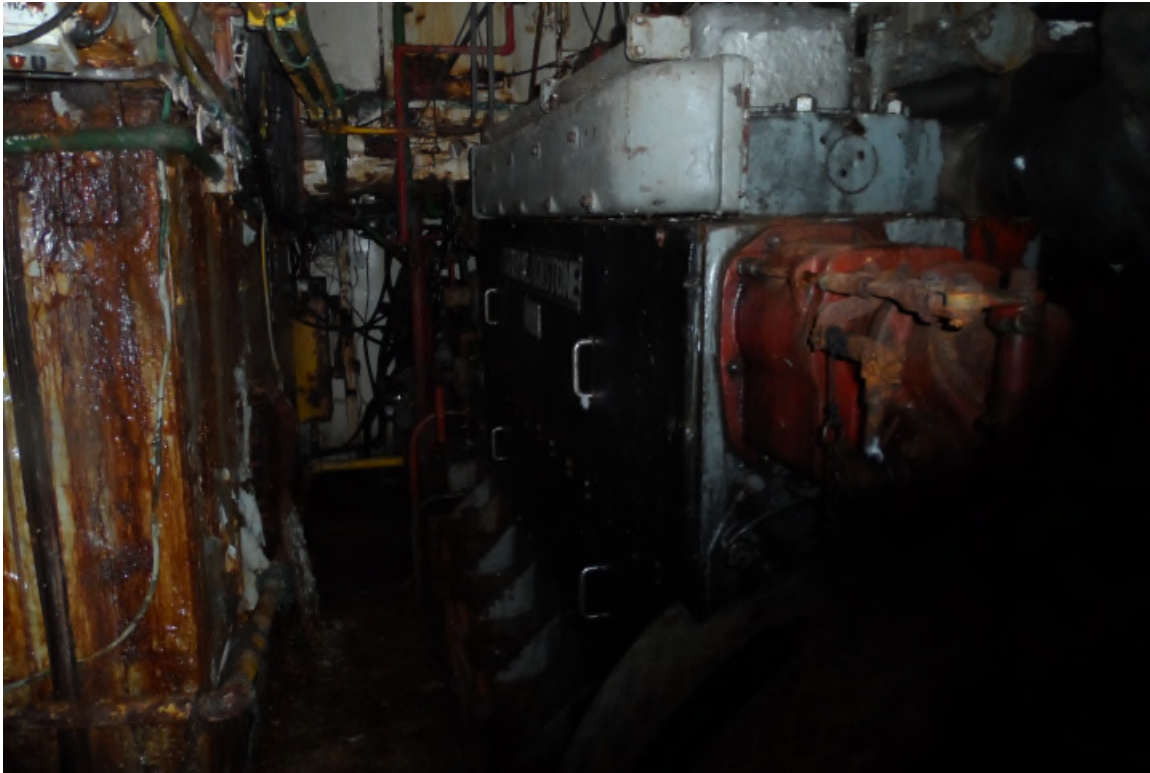
Engine Room 7.JPG
