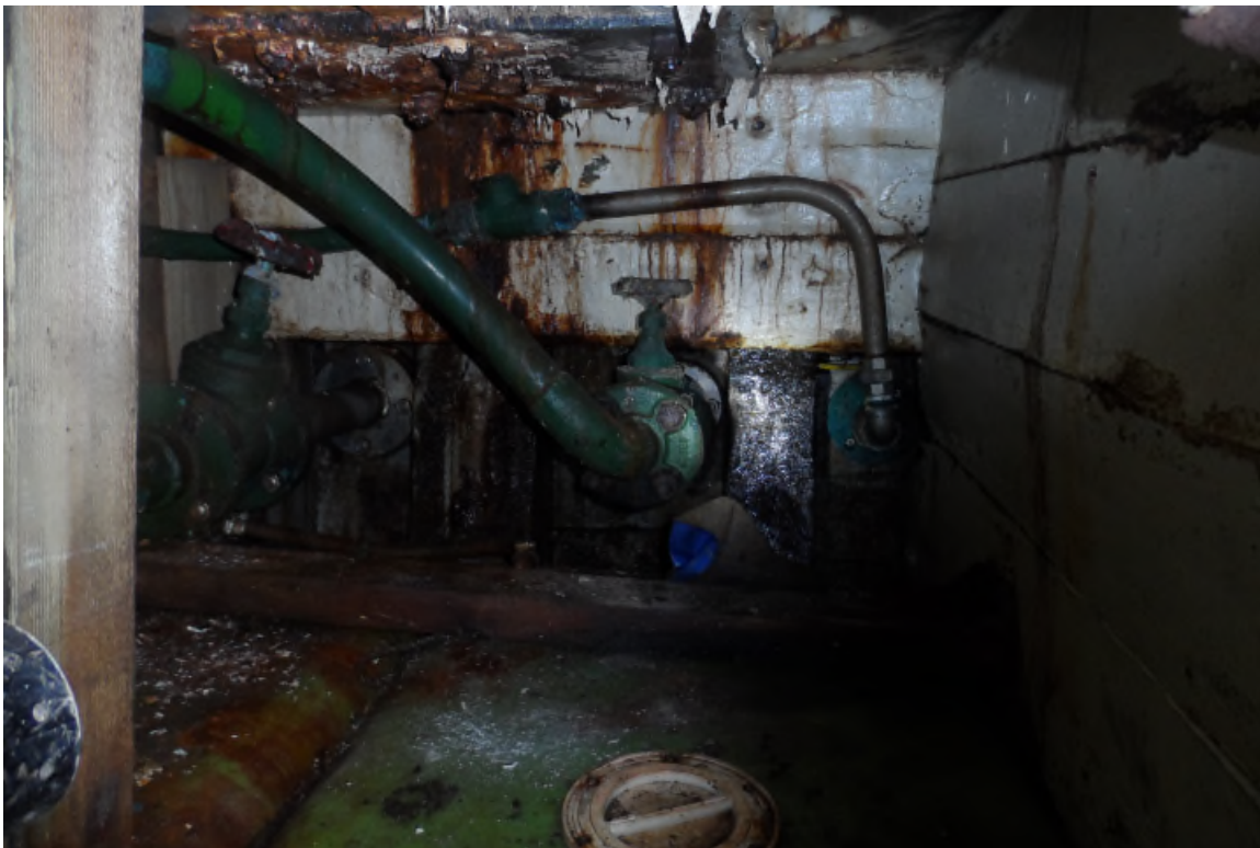
Engine Room 8.JPG
