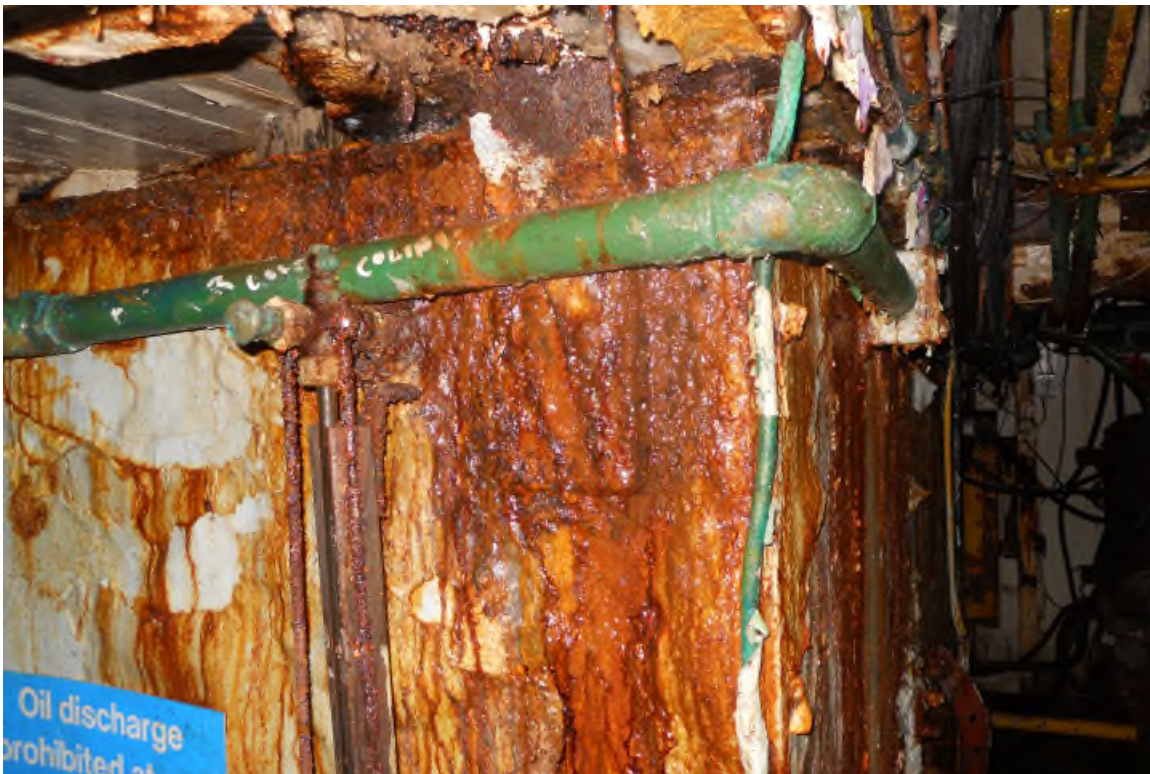
Engine Room 4.JPG
