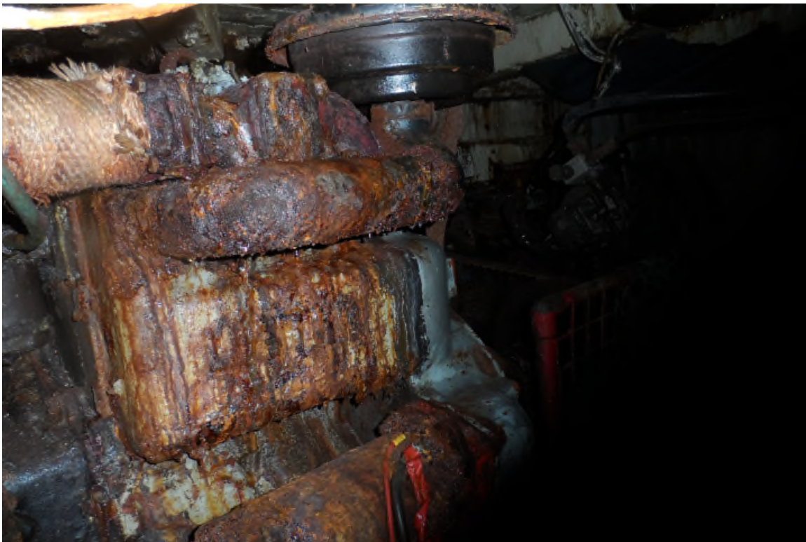
Engine Room 6.JPG
