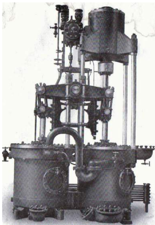
The Weir Dual air pump, Express type, c 1913
