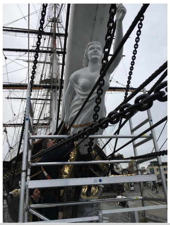
The next stage for Nannie, is to help setup scaffolding to support the figure while she is lowered and measured. This it to double check the shape of the figure head of course, but also to check how she sits and is bolted to the boat.
