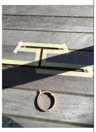
This is much the same as caulking the hull, something I did back in February, but there are a few small changes. Here I was working on the Liverpool house roof deck, which had its own unique caulk to the rest of the deck. This is because traditionally it is where the sail maker worked, and white caulk was used to avoid any black marks being left on the sails as they were being repaired. We use a like for like modern alternative here called white Sikaflex.
