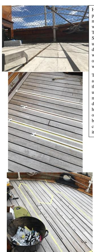
Here on the poop deck, on the portside of the steering gear I did much the same although this caulk was the same used on the main deck. This being the Teakdecking Systems SIS440. After a bit of rain, I had to use the heat gun to speed up the drying process for the seam. This works by applying extra heat to draw out all the water from the exposed wood.
