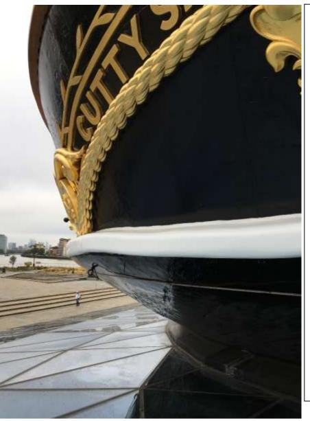
One of the main tasks that we got on with was the painting of the entire hull. We started sanding or keying the portside of the hull from the bow stem down to the stern rudder. Using the Makita palm sanders over the course of a couple days we managed to complete one side. Next came the painting which when distributed among the team in old grime tubs, meant we covered a lot of ground quickly and finished the first coat with in three days.
