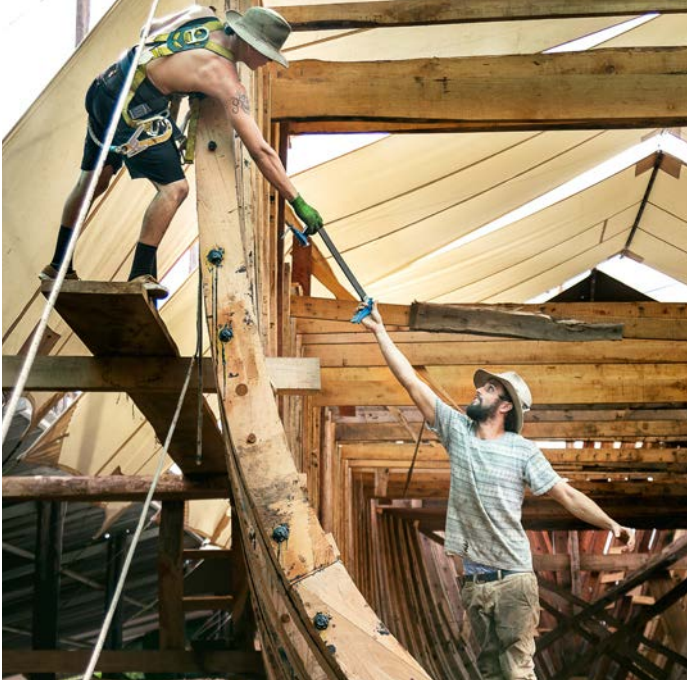
Breidy and Julian raising a frame, by Jeremy Starn.
