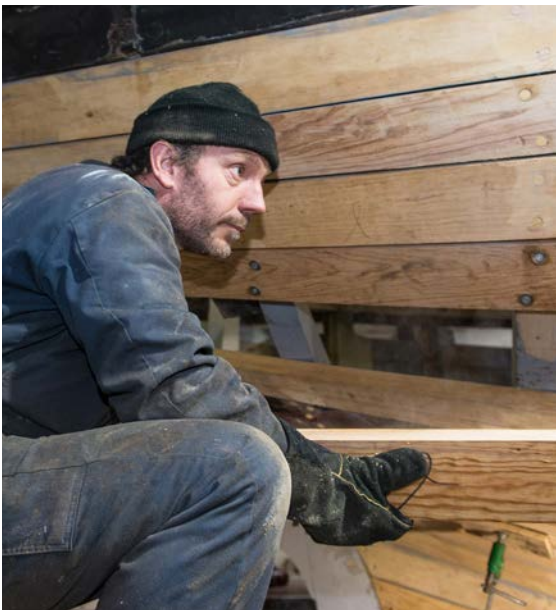
Fitting the shutter plank, by tbc.
