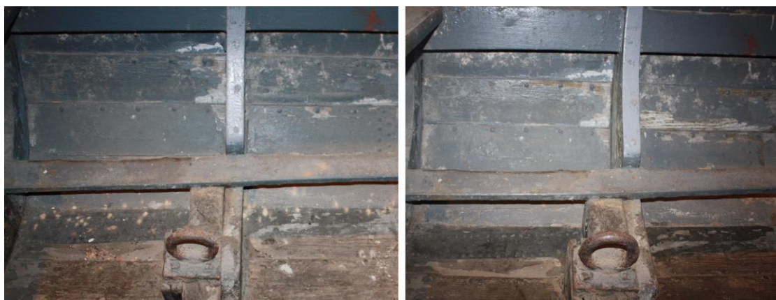
(JUBILEE: Before and After pic of conservation work.)
