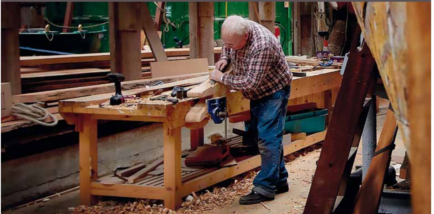
Repairs can be carried out on the vessel or in a workshop or boatyard setting. Photograph by Granville Davies.
