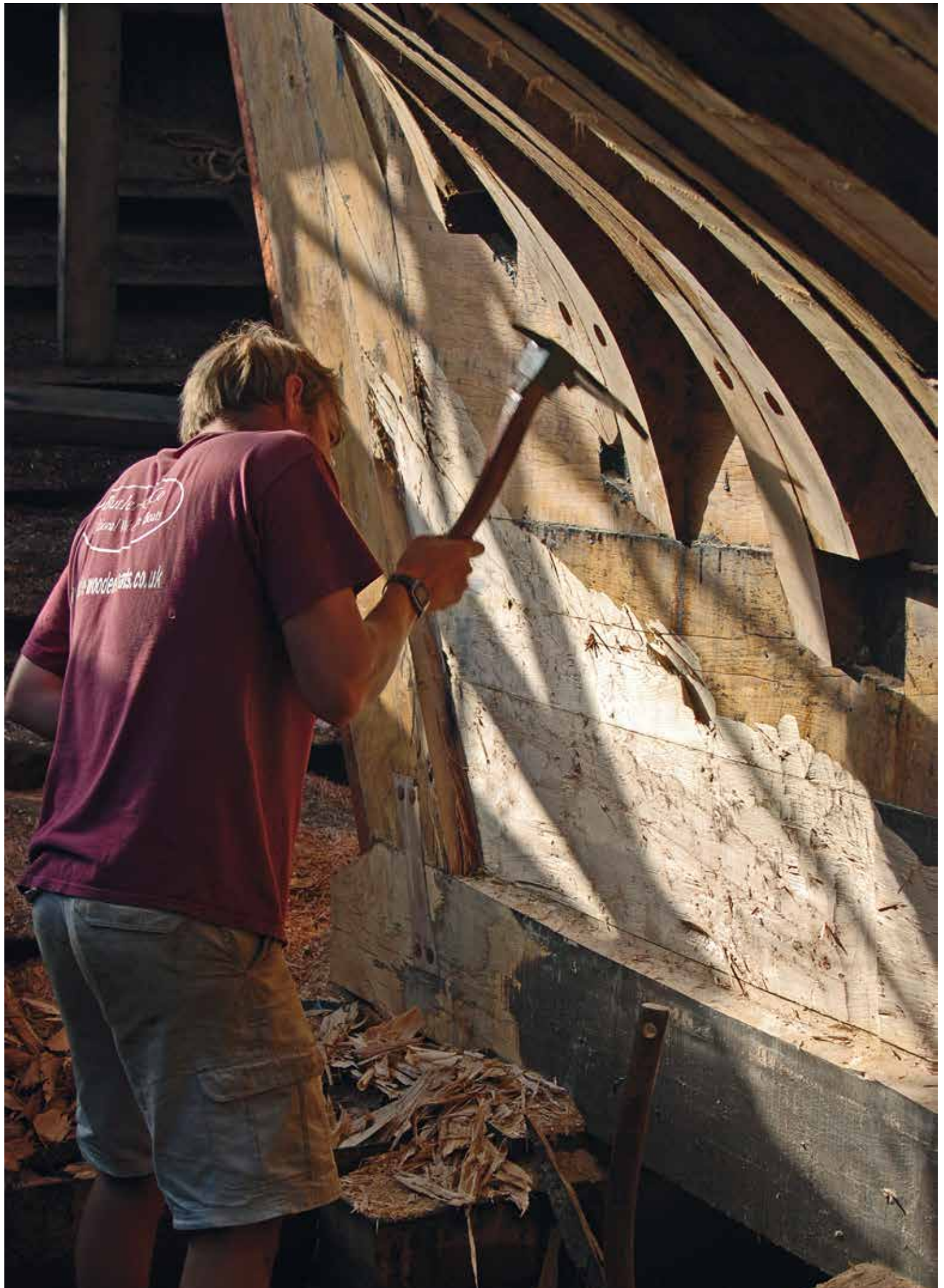
Traditional shipwrights used a range of hand tools including the adze. Photograph by Andy Murray.
