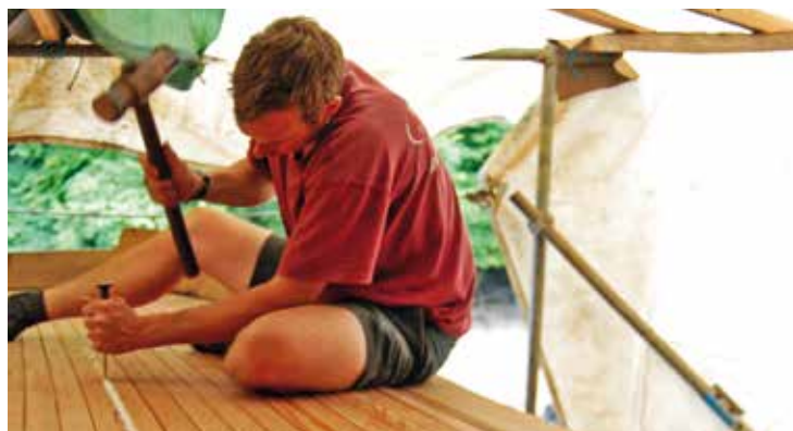
Caulking the deck using traditional methods. Photograph by Rodrick Rigden.
