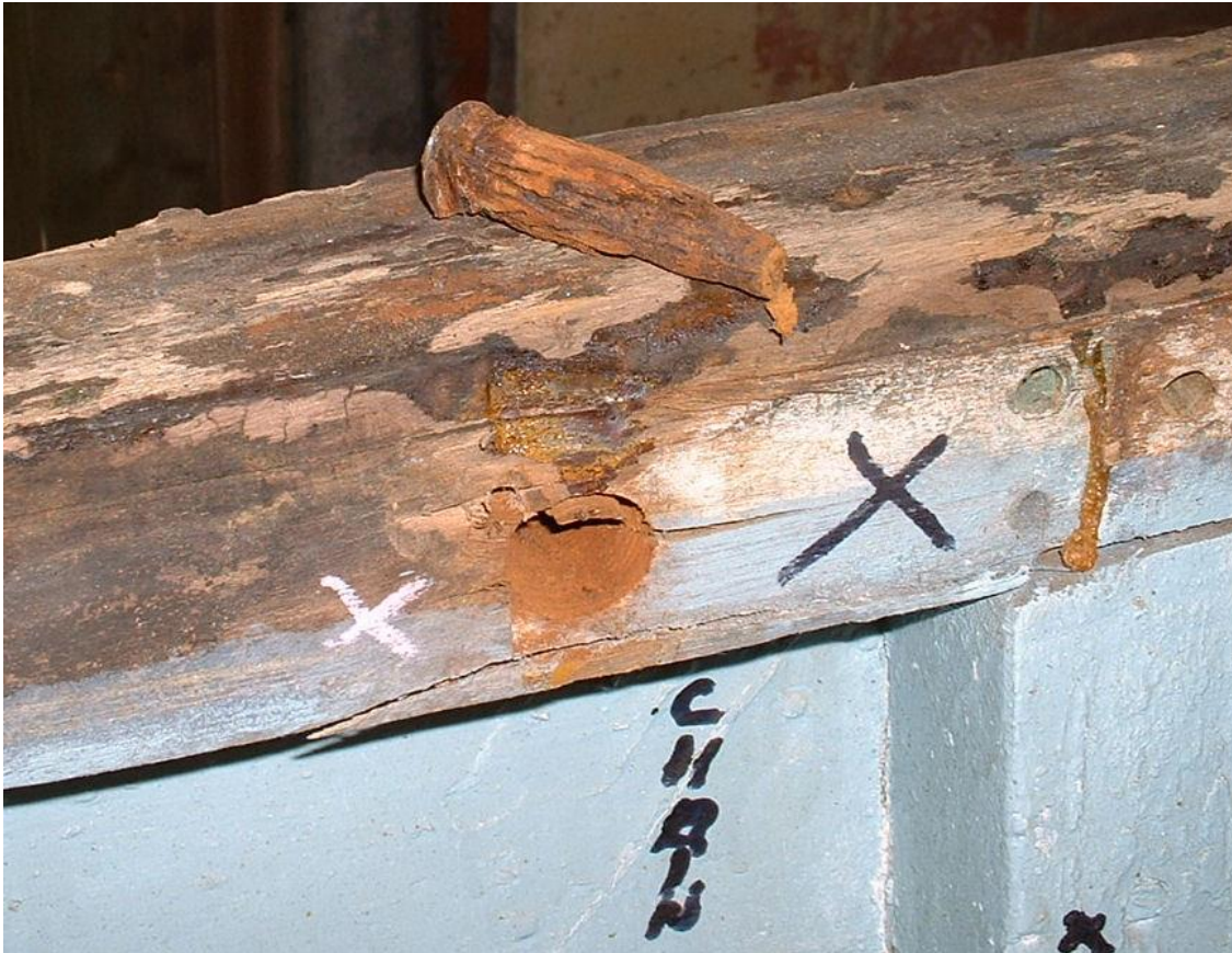
Fig.8b Corroded wrought iron fastening withdrawn
