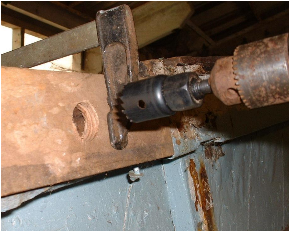
Fig.8a Core of timber around the corroded wrought iron fastening bored out with the help of a plywood guide.
