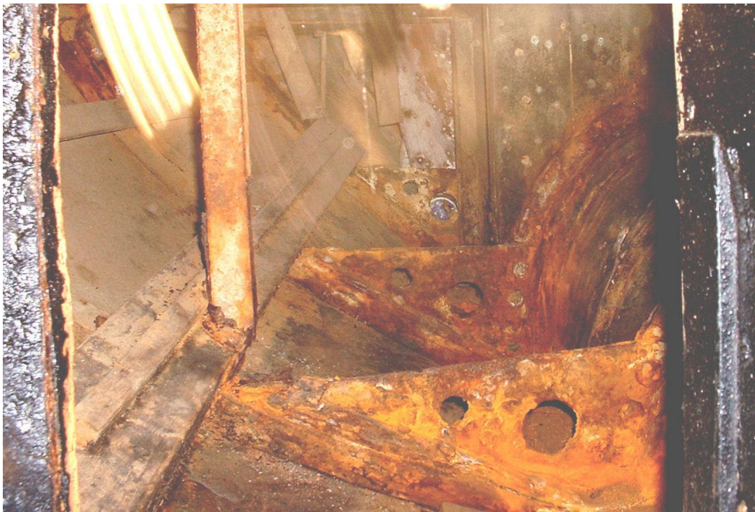
Fig.3 View of the mild steel floors on the starboard side of the propeller tunnel. Most of these floors disintegrated when tapped with a hammer.
