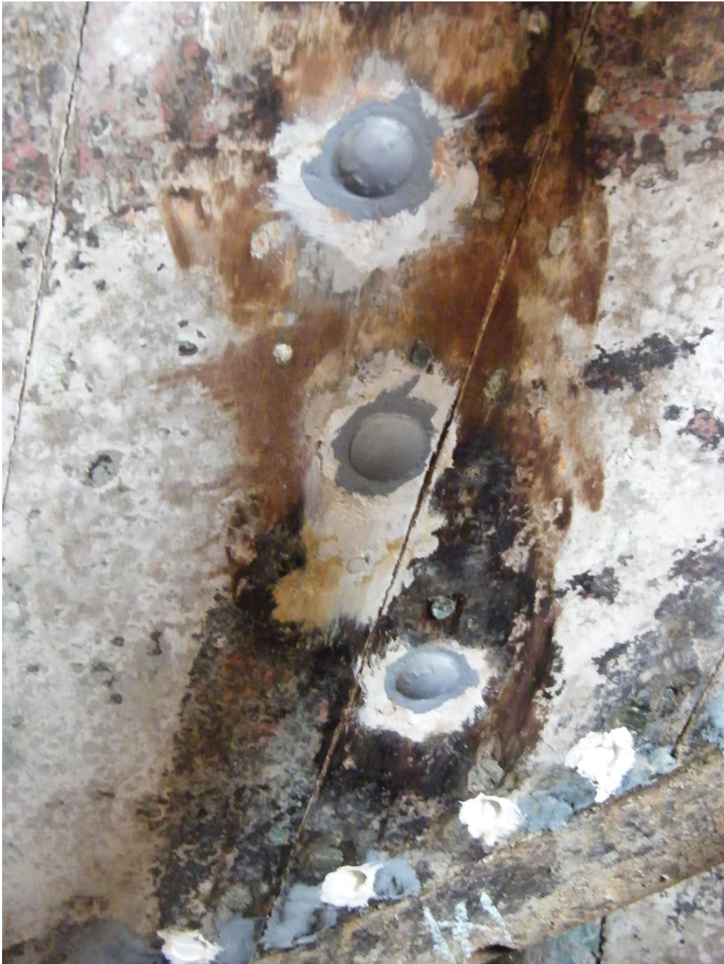
Fig.7d The new fastenings in place. Each bedded down with white lead paste and a twist of caulking cotton under the head.
