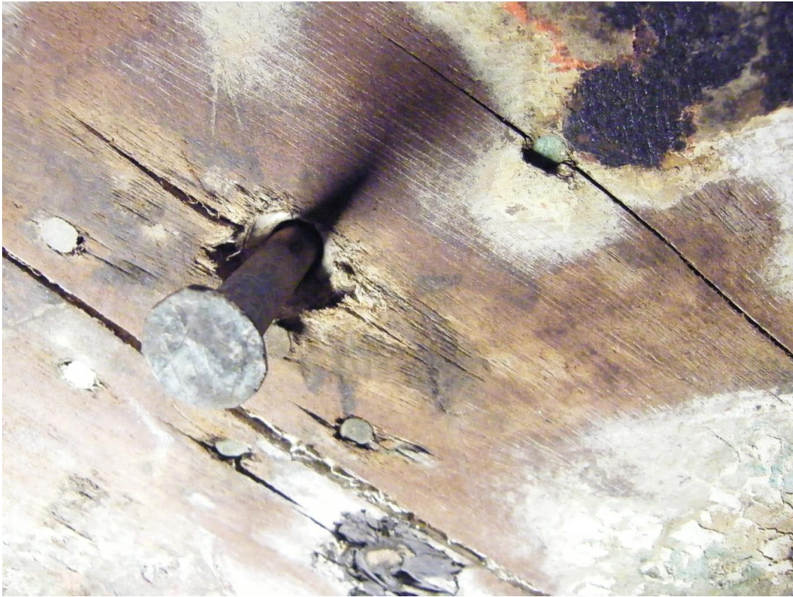
Fig.7a A close-up view of one of the 3/8" diameter floor fastenings being withdrawn, showing the secondary effect of bi-metallic corrosion.
