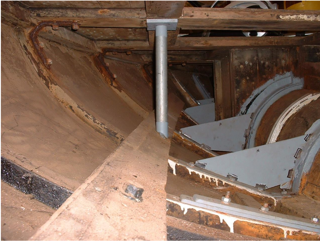
Fig.5 The floors and deck support shown in Fig.3 now removed and replaced with mild steel plate coated with epoxy primer. The threaded end of the new galvanised bolts can be seen. Once the new plates have been welded to the original remaining sections around the tunnel, they will again receive numerous coatings of epoxy primer, undercoat and topcoat.
