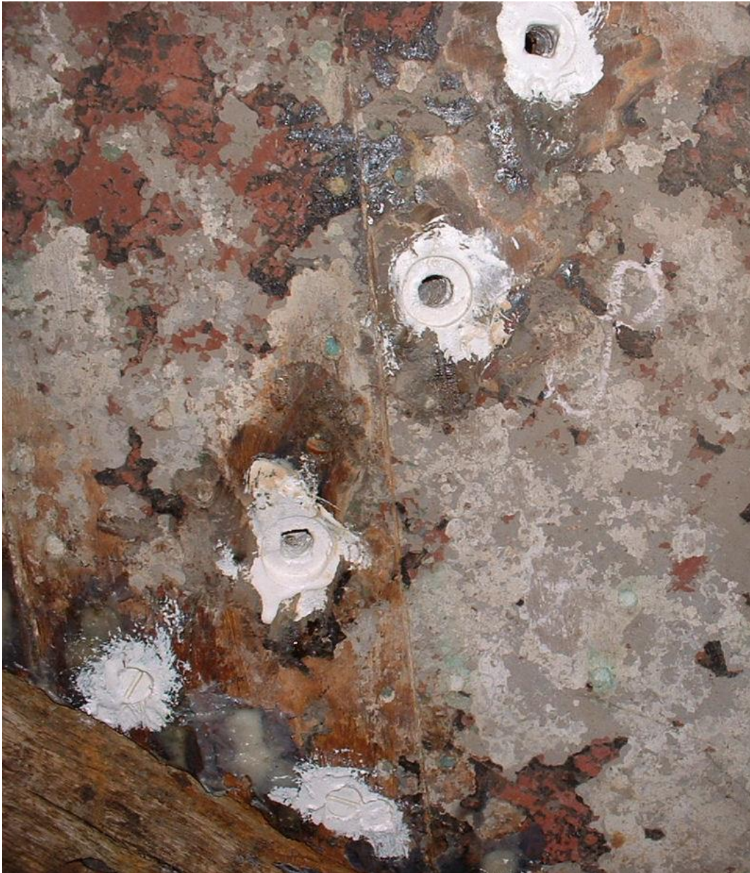
Fig.7c The floor holes prepared to accept the new galvanized coach bolts. To ensure the bolt heads have a good seating, the area under each head has been flattened off using a modified flat drill bit with a central guide having the same diameter as the fastening.
