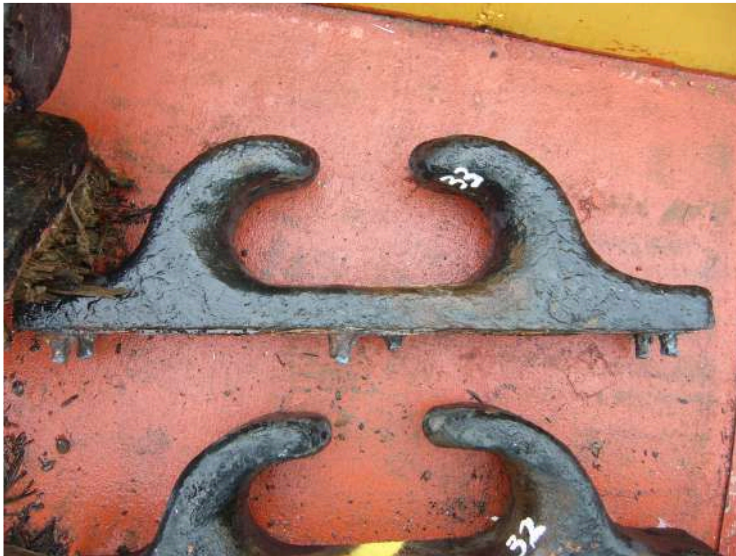
Cleats removed for reuse, note numbering (W. Davies)
